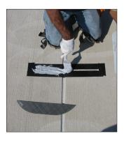
Applying epoxy paste to slot
