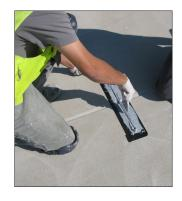
Inserting biscuit in slot
