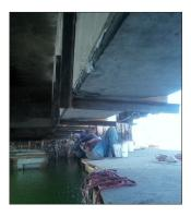
After CFRP plate is applied
