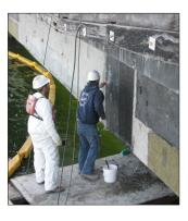
Applying CFRP fabric for shear strengthening
