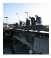
CFRP plate lowering for application
