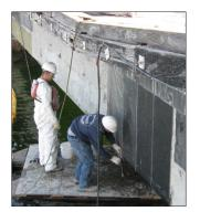
Applying CFRP fabric for shear strengthening
